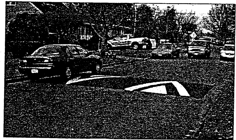
SPEED BUMP DETAIL GAP FOR BIKE (NTS)
