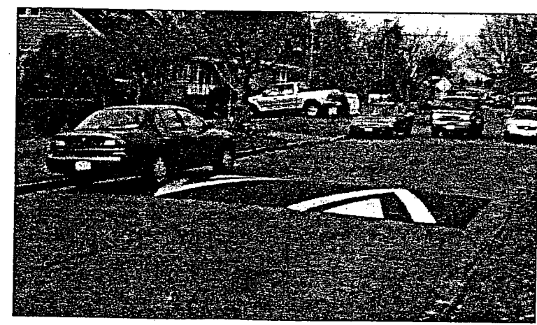
SPEED BUMP DETAIL GAP FOR BIKE (NTS)
