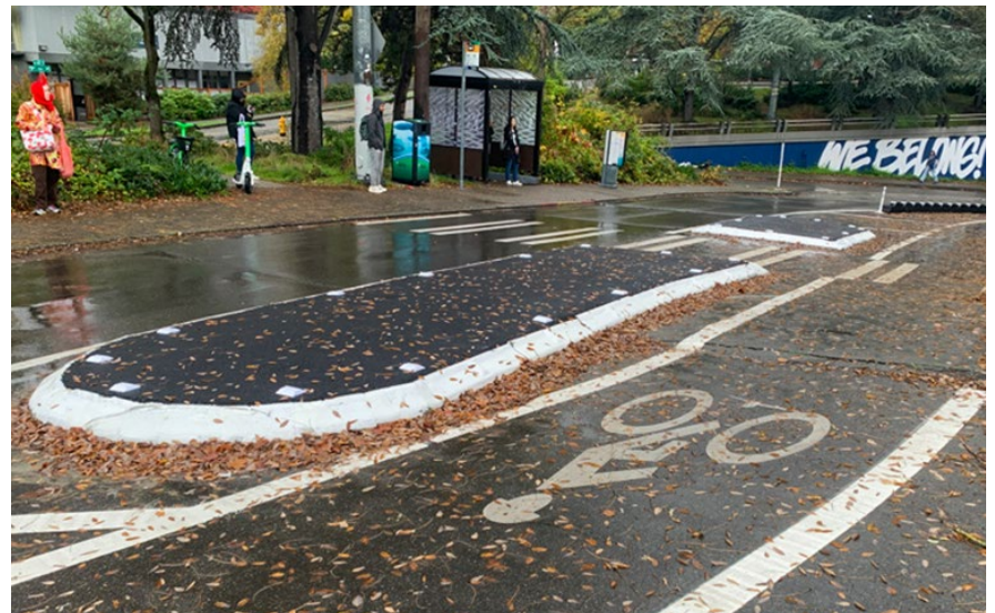
Along NE Campus Parkway, a new type of bike lane barrier made of upcycled tires. Nearby, there is a new asphalt median to separate riders from traffic.
