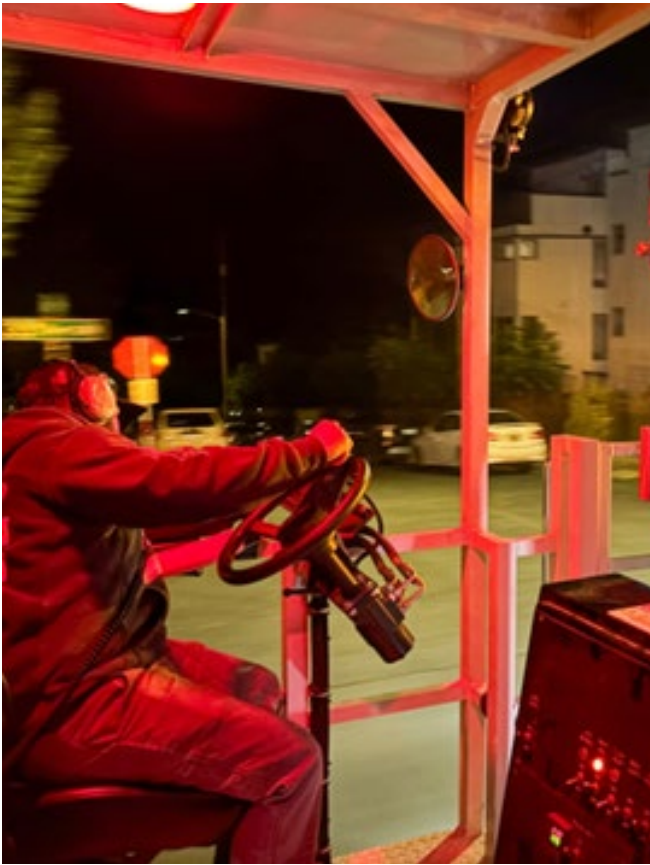
SDOT crews remarking arterial lane-miles.
