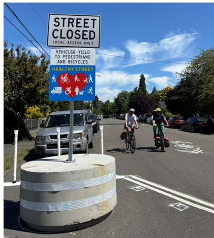
Georgetown Healthy Street and Neighborhood Greenway, which includes elements for safety and traffic calming such as speed humps, Healthy Street signs, concrete sign bases, concrete planters, and painted curb bulbs with flexible posts at intersections. The Healthy Street will be connected to a larger network of Healthy Streets and Neighborhood Greenways.
