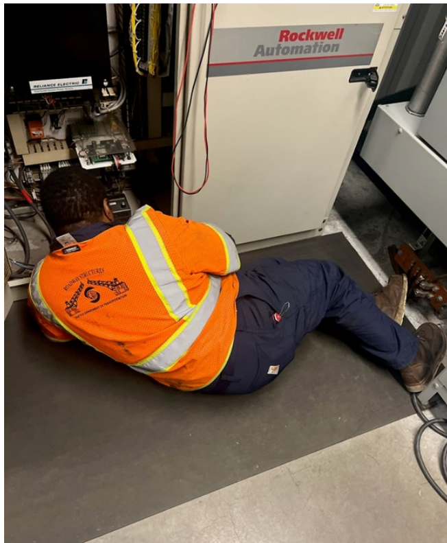
Performing electrical preventative maintenance on the Ballard Bridge.
