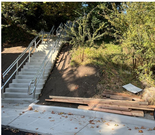
Repaired stairway on S Brandon St.
