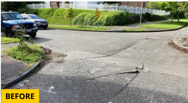
Before and after a repaving project on 16th Ave S. We removed damaged concrete panels and patched with full-depth asphalt.
