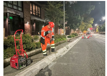
SDOT crews installing new better bike lane barriers on E Yesler Way.
