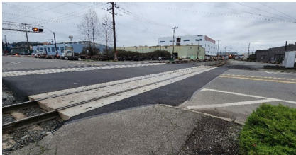
Repaired crossing surface at S Hanford St
