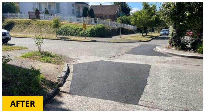
Before and after a repaving project on 16th Ave S. We removed damaged concrete panels and patched with full-depth asphalt.
