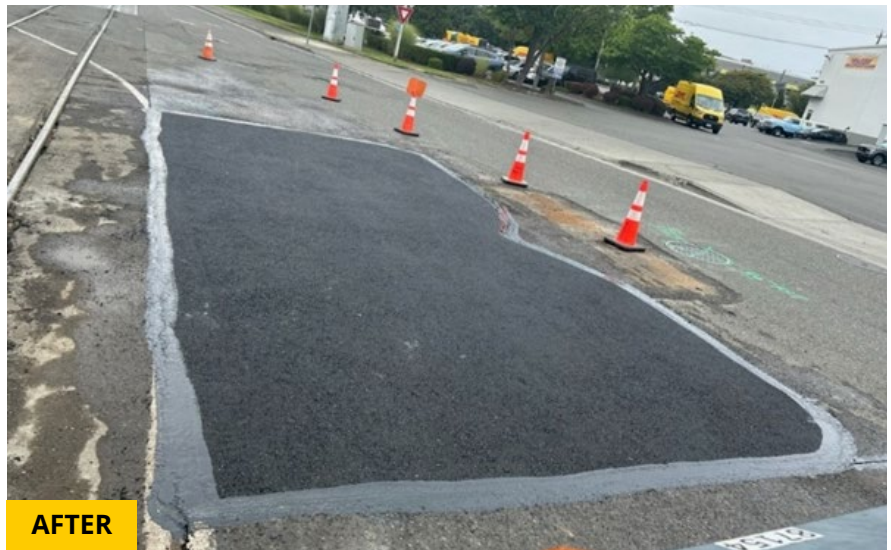
Before and after sinkhole repair at Diagonal Ave S/Colorado Ave S/ S Oregon St.
