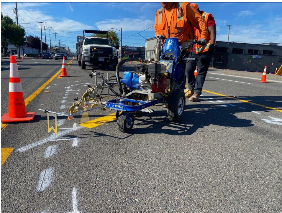
Installing a median on 4th Ave S and S Massachusetts St.
