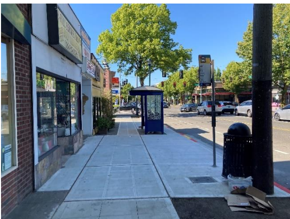
Repaired and improved bus zone on California Ave SW and Admiral Way N.
