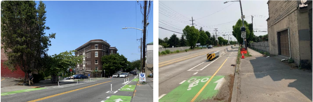
Protected bike lane on Melrose Ave E (left) and protected bike lane on West Marginal Way SW (right).
