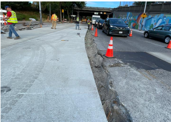
Repaving on N 46th St in progress.
