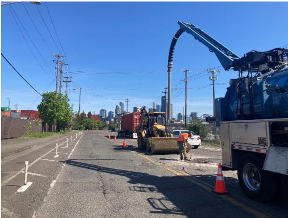
Potholing for a water main on East Marginal Way S.
