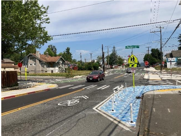
Part of the 51st Ave S and Renton Ave S Traffic Safety Enhancements project (left); new curb bulbs and ramps, concrete panel replacement as part of the Andover and Dakota Pedestrian Safety Enhancements project (right).
