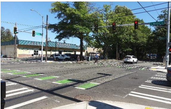
Improved crossings on Rainier Ave S as part of Route 7 work.
