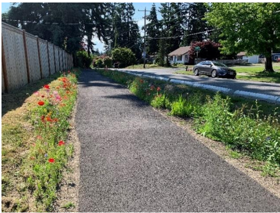
New walkway on NW 132nd St in progress.
