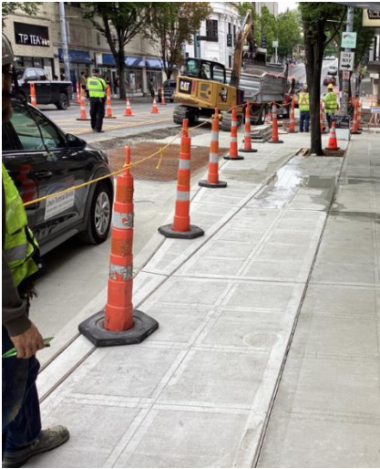
Improving sidewalks as part of the Route 44 project.
