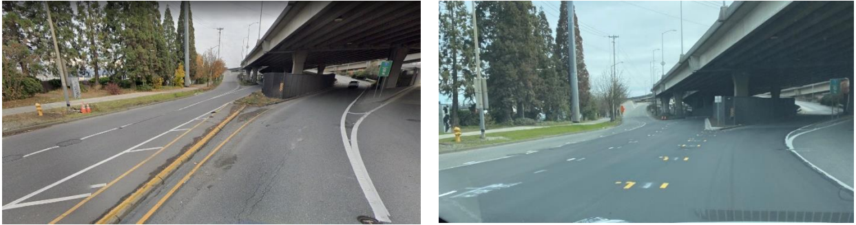
Before (left) and after (right) lane extension on S Spokane St at SB SR-99 off-ramp.
