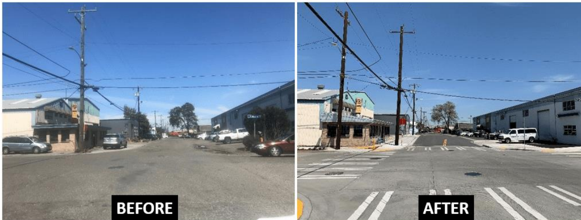
One of numerous areas improved as part of this project: 5th Ave S & S Holden St. This image shows the area during a flood.
