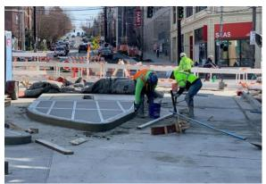
As part of the Madison RapidRide G Line project, we have installed foundations for new bus shelters (shown here on Union St for the Route 2 bus).
