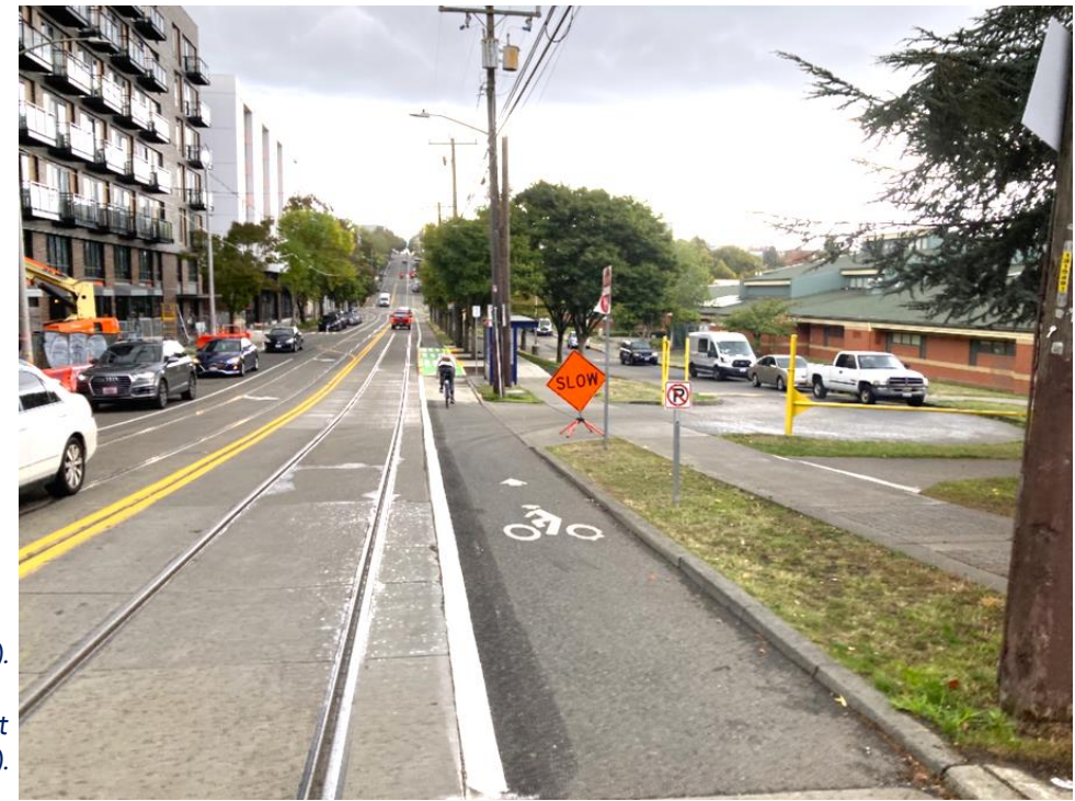
Delineators between railroad lines on S Spokane St (top).
