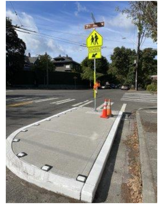
Before (left) and after (right) installation of new curb bulb and signs near Thornton Creek Elementary School.
