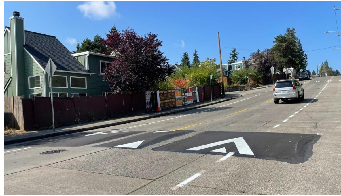
Program 2 – Speed humps to slow vehicle speeds near Chief Sealth High School and Denny International Middle School.
