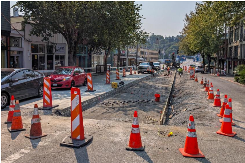
As part of the Route 40 project, repaving in Fremont (left) and crews finish concrete for the new sidewalk west of the bus stop area on N 35th St, east of Fremont Ave N (right).
