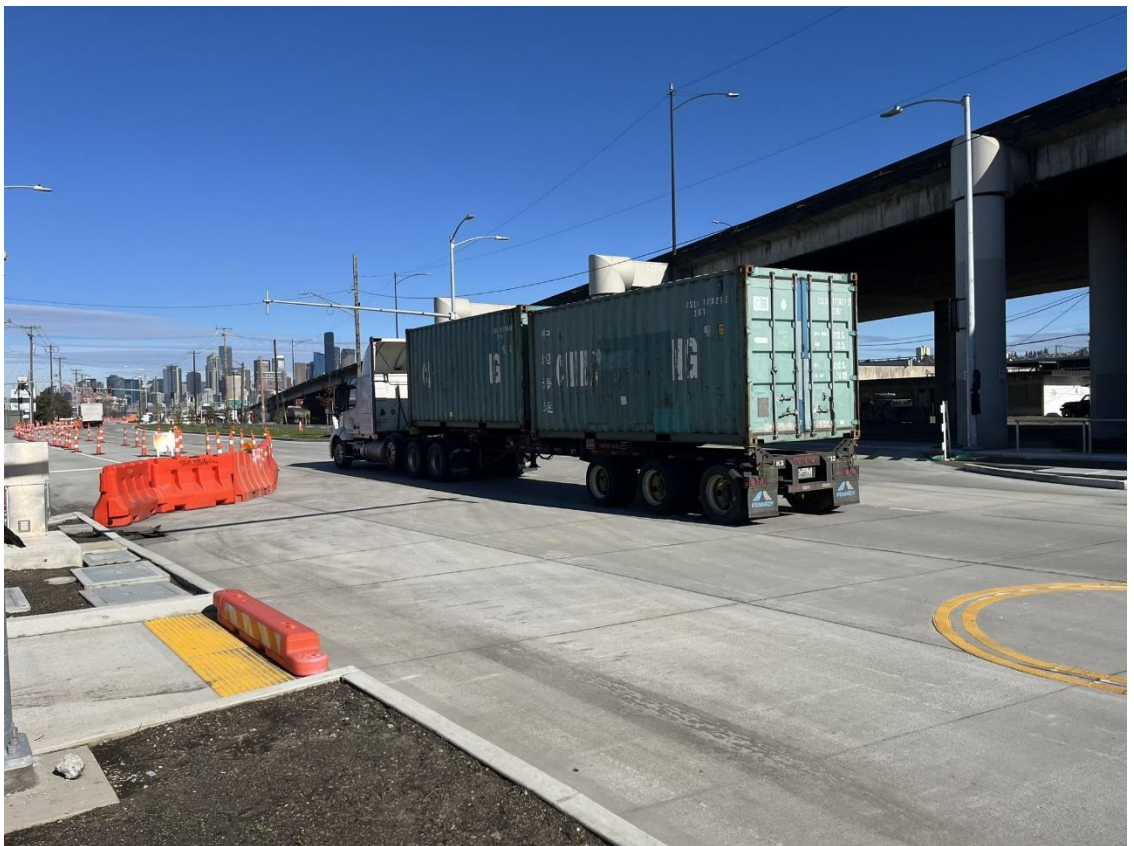
A large freight truck travels north on the newly repaved E Marginal Way S.
