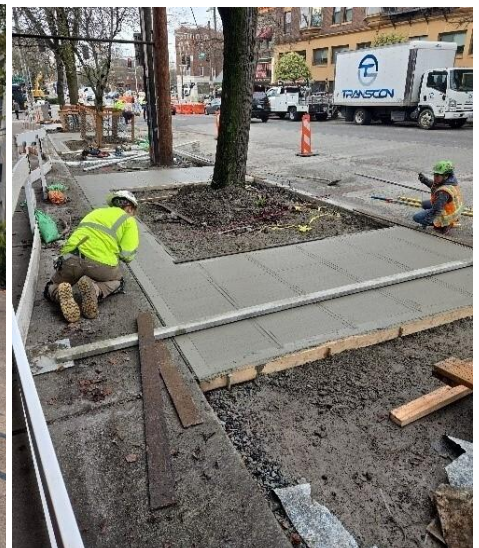
As part of the Route 40 project, repaving in Fremont (left) and crews finish concrete for the new sidewalk west of the bus stop area on N 35th St, east of Fremont Ave N (right).
