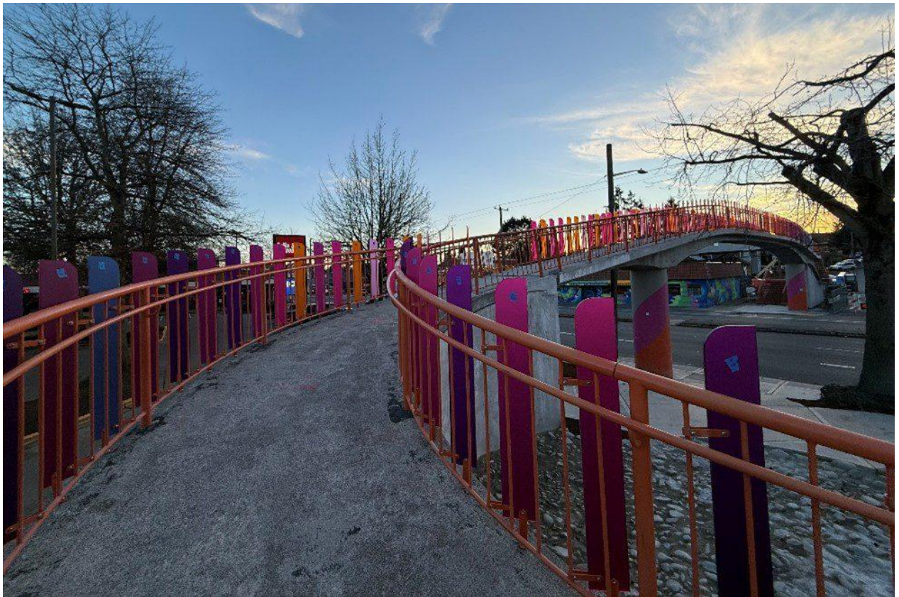
N 102nd & Aurora Pedestrian Bridge near Licton Springs
