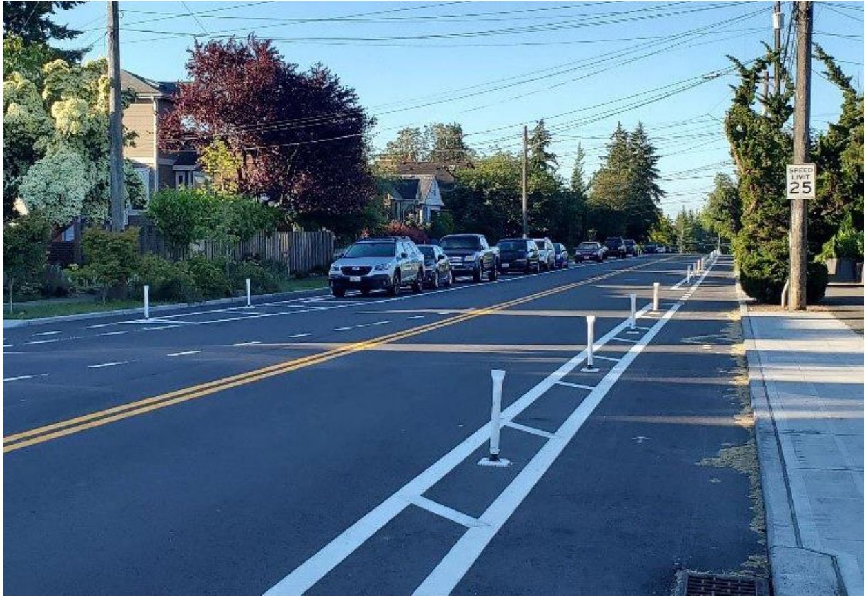
Program 9 – Repaving on 15th Ave NE. We also rechannelized the street, making room for bike lanes going in both directions.
