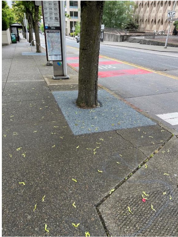
Program 21 – Red bus lane on Pine St (left); Tree pit on 5th Ave filled for bus passenger comfort and safety (right).
