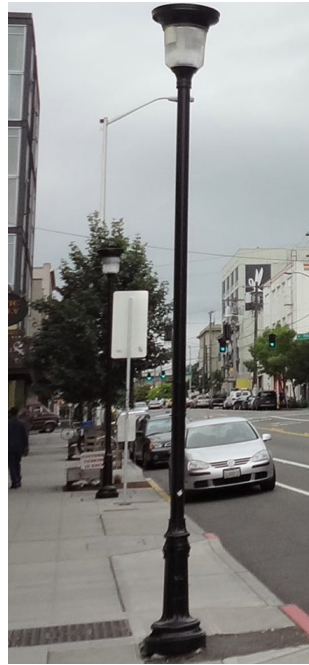
Image 5: Light pole with post-top light
