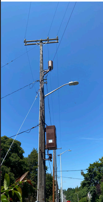
Image 2: Side-mount canister antenna and equipment cabinet on a wood pole
