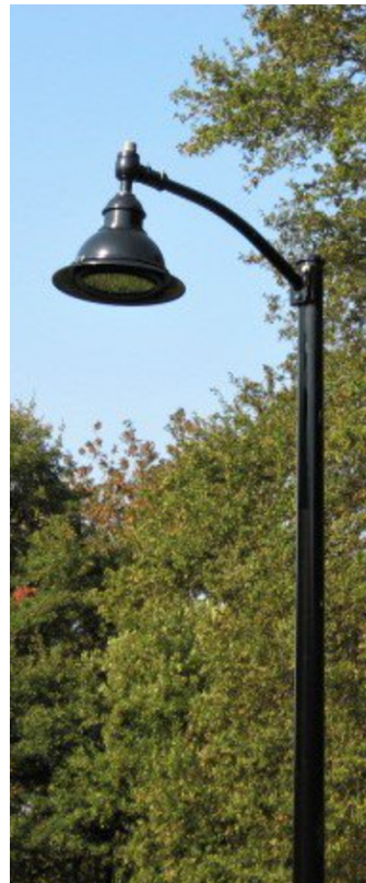
Image 10: Decorative light pole along Lake Washington Blvd
