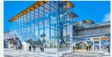
Station designed with maximum transparency and clear sightlines to elevators, platforms, and destinations. Wood on the canopies provides a focal point and adds warmth and texture.
