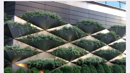
Green walls with integrated planters and irrigation breaks up the scale of a large wall while ensuring the long-term health and success of the plantings.
