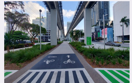
A bike path under the guideway enhances community connections and mobility.
