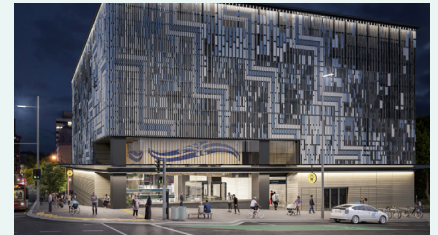
A blank facade is designed with a pattern of basalt and glass inserts that represent local Indigenous deities and heritage, creating a focal point and reducing the visual scale of the facade.
