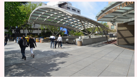
Wide sidewalks for pedestrian at station frontage
