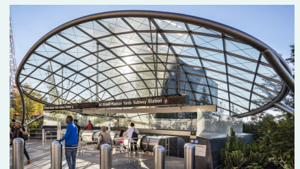
Iconic canopy creates a legible and welcoming entry while maximizing daylight to the levels below.
