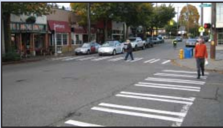
Crosswalks repainted at 15th Ave E and E Republican St.
