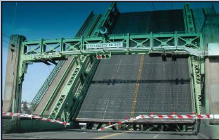
Maintenance and repair work done on the University Bridge
