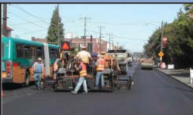
New street paving in Northeast Seattle.
