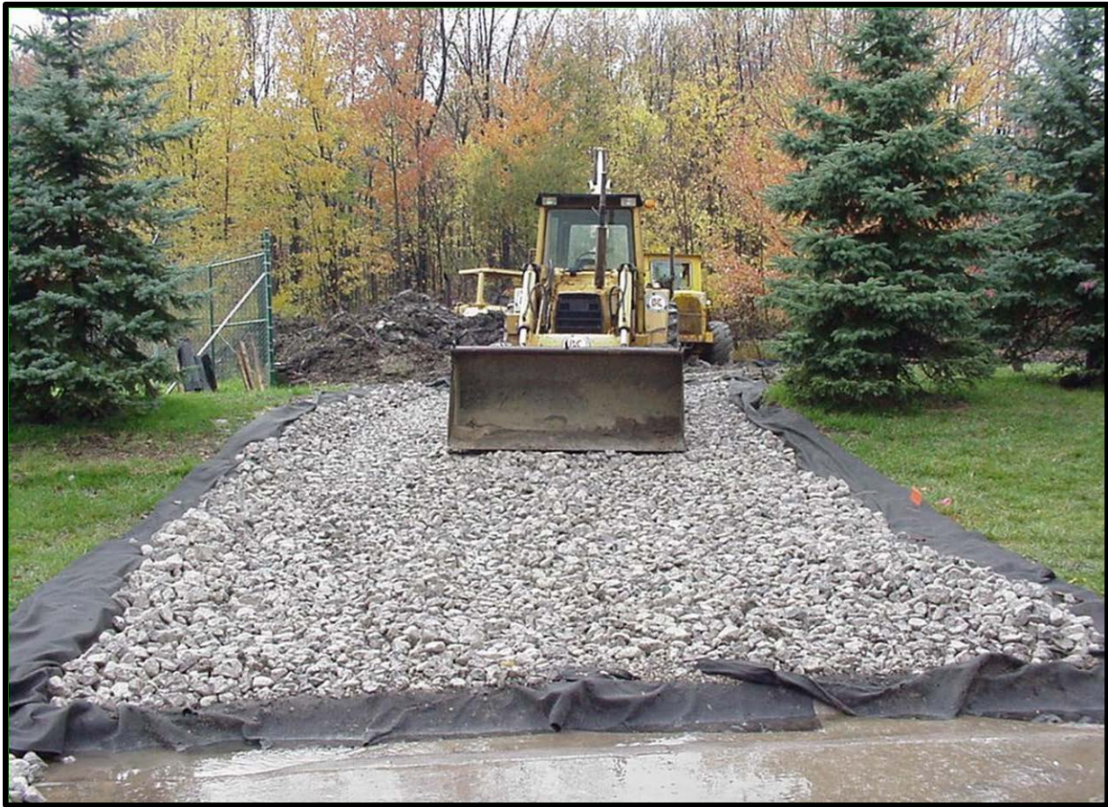
Figure 6. Stabilized Construction Entrance.
