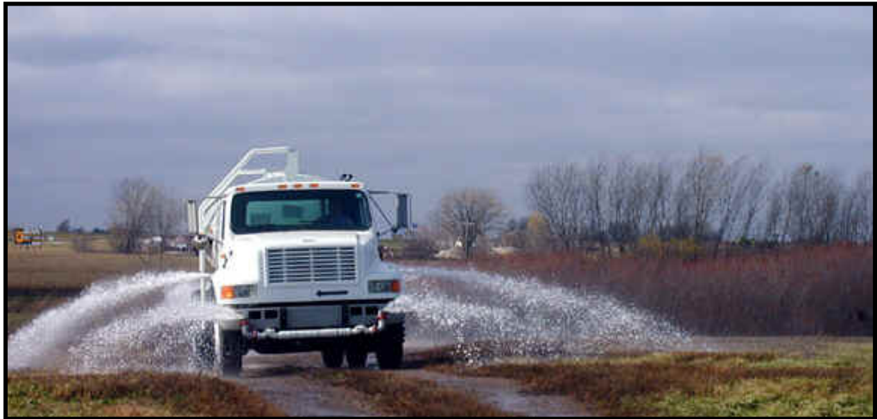
Figure 11. Using a Water Truck for Dust Control.
