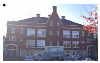
This building is irregular in terms of its shape and window openings. The brick façade will need to be connected to the structural brick behind it. Because this building is a school, and thus a critical structure, additional requirements may be placed because of its use. Additional considerations that may impact seismic considerations include the soil type for liquefaction hazards and foundation elements.
