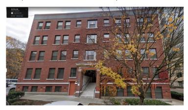
This building was of regular shape, had equal size windows, continuous load paths. The number of window openings can determine the type of upgrades that need to be done inside the building. The building is U shaped and has a smaller floor diaphragm, providing opportunity to build additional lateral support which serves to increase seismic resistance.
