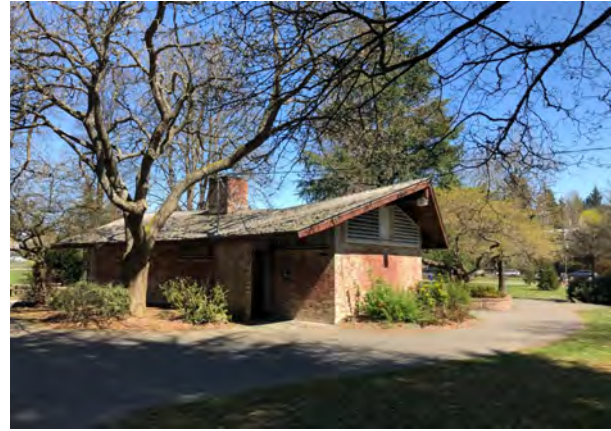
Improve accessible entrance from NE 70 th St. Match grade to sidewalk. Regrade and replace asphalt with concrete walk to restrooms.
