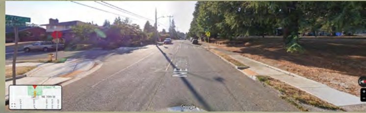
COMPLIANT CURB RAMP AT NE 70 TH ST & 44 TH AVE NE
