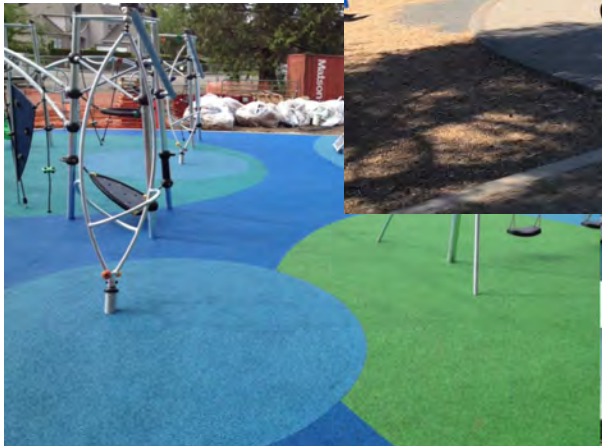
Use pour-in-place safety surfacing for accessible surfacing. Use engineer wood fiber for swing area except for accessible swing.
