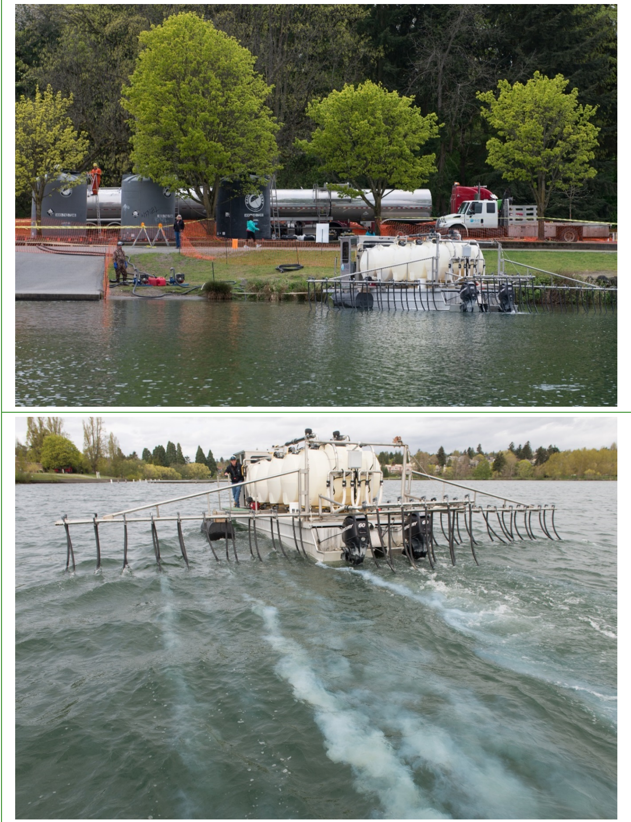
Figure 3. Staging Area and Application Photographs for the 2016 Green Lake Alum Treatment.
