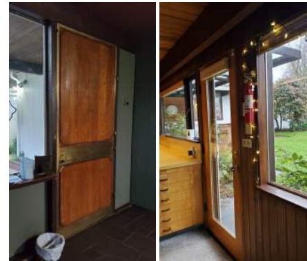
Existing Wood Entry Doors
