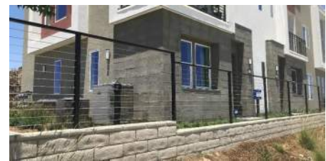
Example of cable guardrail system
