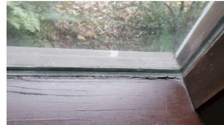
Existing Single-Pane Glazing
