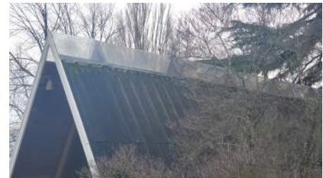
Existing Plastic-Glazed Ridge Skylight
