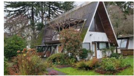
Accessible Exterior Approach
