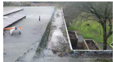
Existing Low-Slope Roof Drainage
