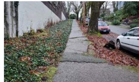
South Retaining Wall at E. Prospect
