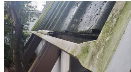
Existing A-Frame Roof Gutter
