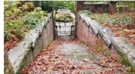
West Site Access Stair
