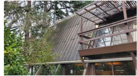
Existing “A-Frame” Roof Portion
