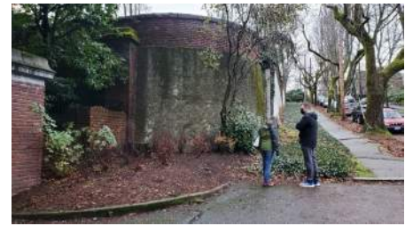
Wall from SW Corner of Bullitt Estate
