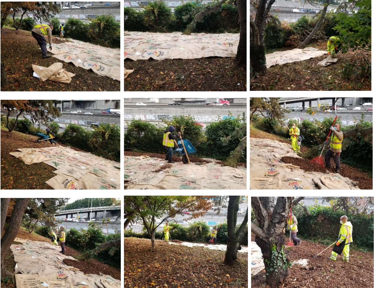
Laying burlap, delivering, and spreading mulch
