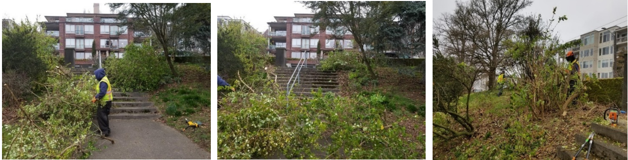
After-Stairway cleared of brush for CPTED
