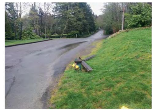
12. Excavate around fire hydrant to provide 2" minimum clearance from the hydrant's flange connection to grade, remove curb stops and provide bollards to protect hydrant per City of Seattle details.
