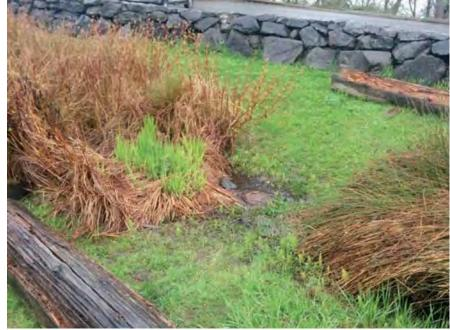
3. Clean and rechannel biofiltration swale located outside the northwest entrance.
