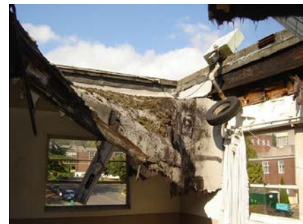
A deteriorating building at Magnuson Park
