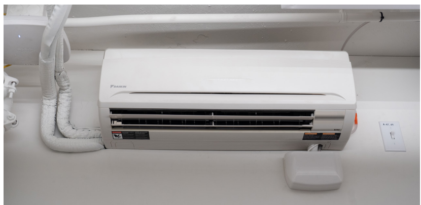
Interior heat pump unit
