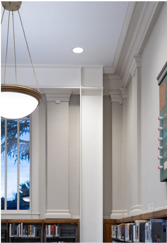
New steel pillars add earthquake protection and blend into the historic architecture
