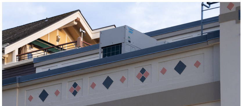
Heat pump condenser on roof
