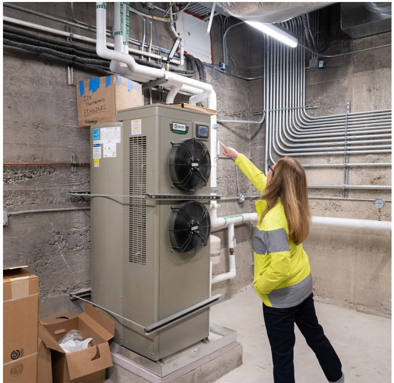
New efficient, electric heat pump water heater
