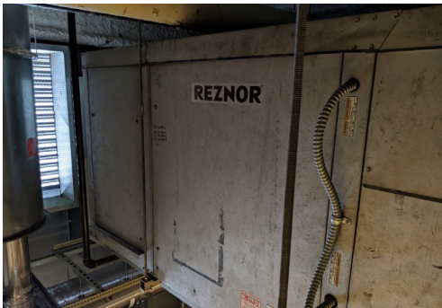
The failing makeup air unit provides ventilation for the building and needs to be replaced soon.
