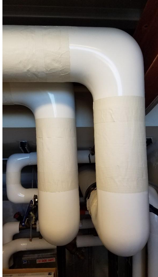
Photo 23. New insulation on piping in penthouse area.
