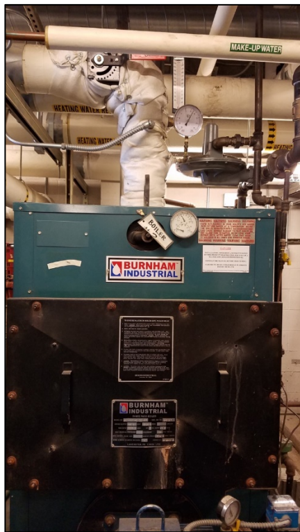
Photo 11. The less efficient non-condensing boiler was carrying the primary load.
