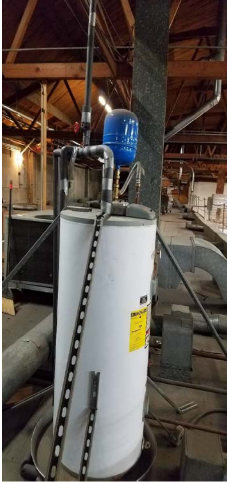
Photo 7. DHW pipe insulation installed March 2019.
