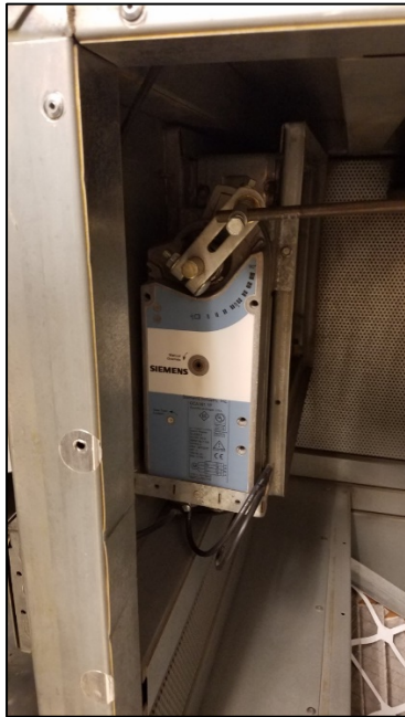
Photo 13. New damper actuator.
