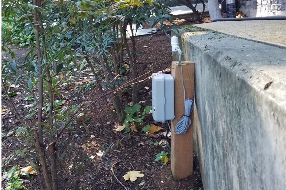
Photo 22. A rain sensor was added to the irrigation system.
