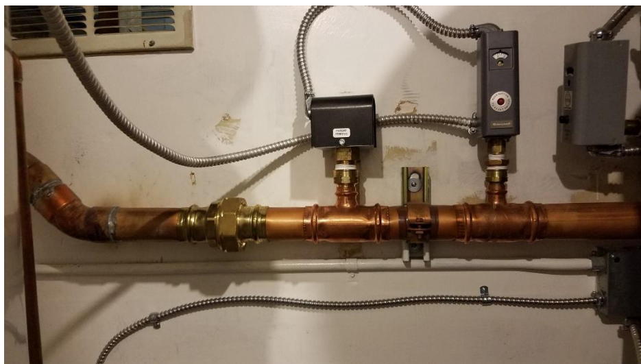
Photo 3. New wiring and plumbing to prevent circulation pump operation when boilers are not firing.
