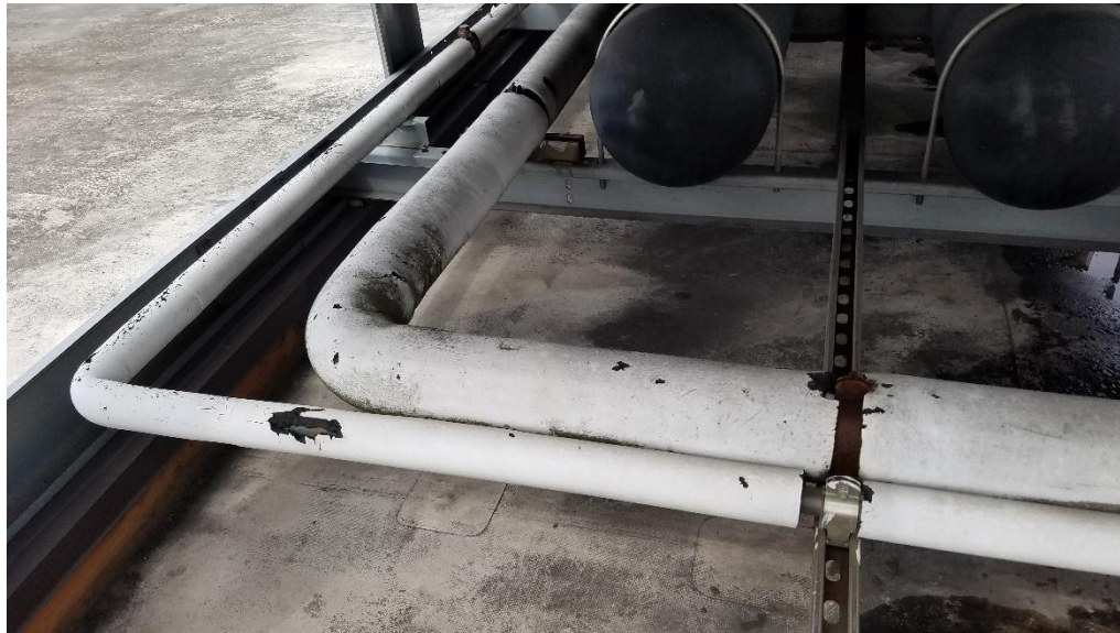
Photo 9. Uncovered insulation had sustained more damage from birds.
