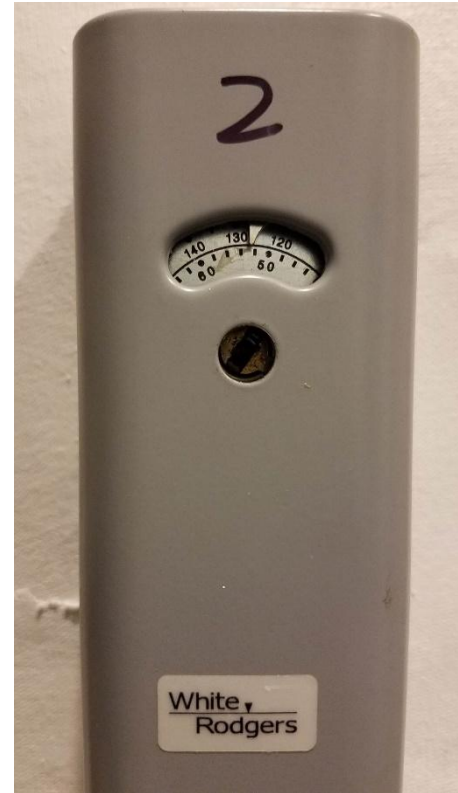
Photo 2. DHW boiler thermostat showing tank temperature.
