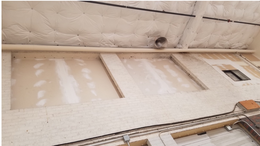
Photo 17. Some windows were filled in and insulated.
