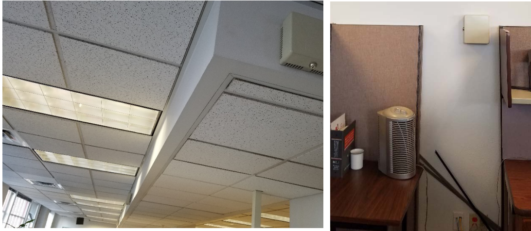
Photo 28. Thermostats were previously located near the ceiling (left) but have been moved to a more accurate location further down the wall (right).
