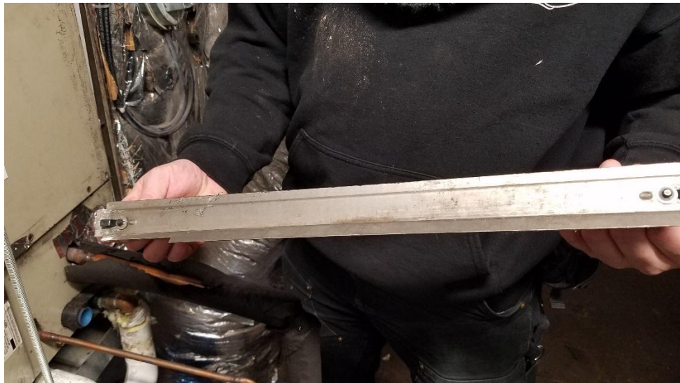
Photo 21. A bracket on the non-functioning filter frame was repaired.
