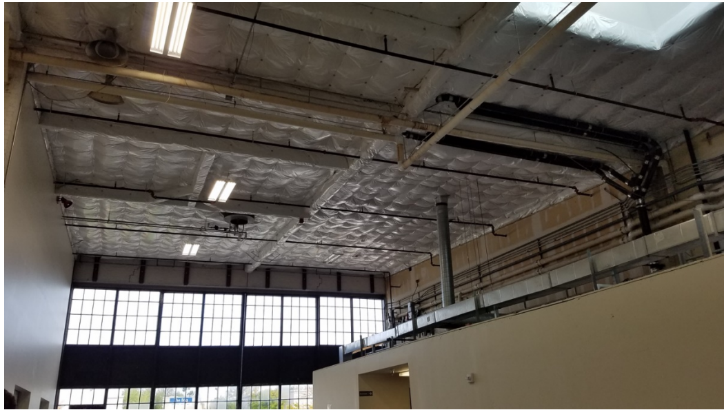
Photo 16. Part of the ceiling was insulated. Note the ductwork to the right that has not been insulated.
