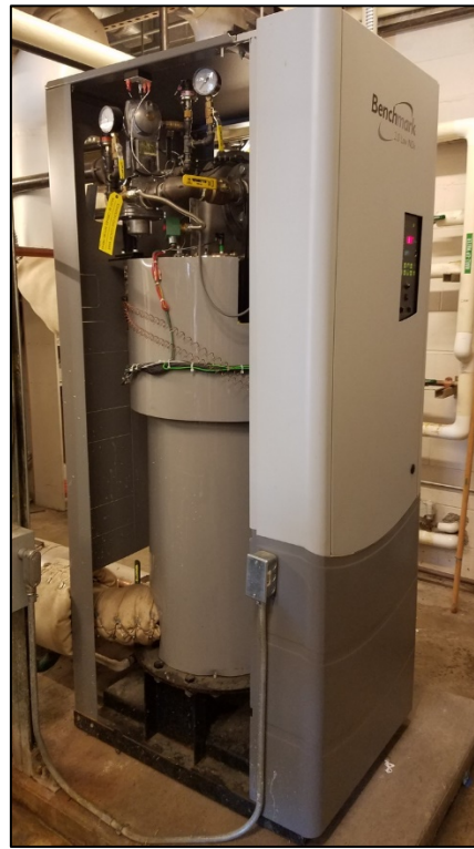
Photo 12. Settings were changed so that the more efficient condensing boiler carries the primary load.
