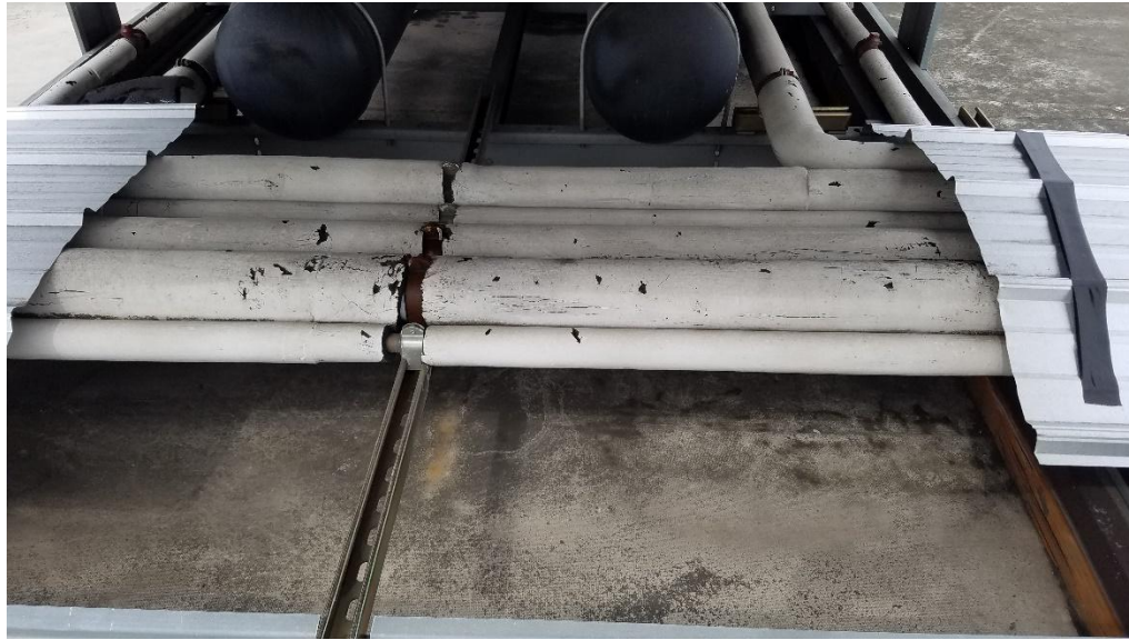
Photo 8. Refrigerant piping on roof was installed, with portions covered to prevent damage from birds.
