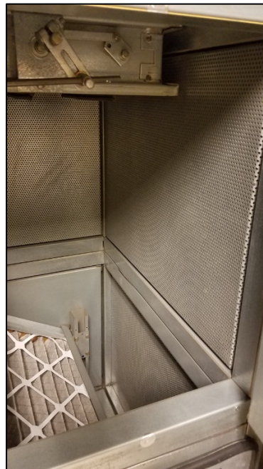
Photo 14. Random inspection of several units indicated filters had been replaced, and coils and plenums had been cleaned.
