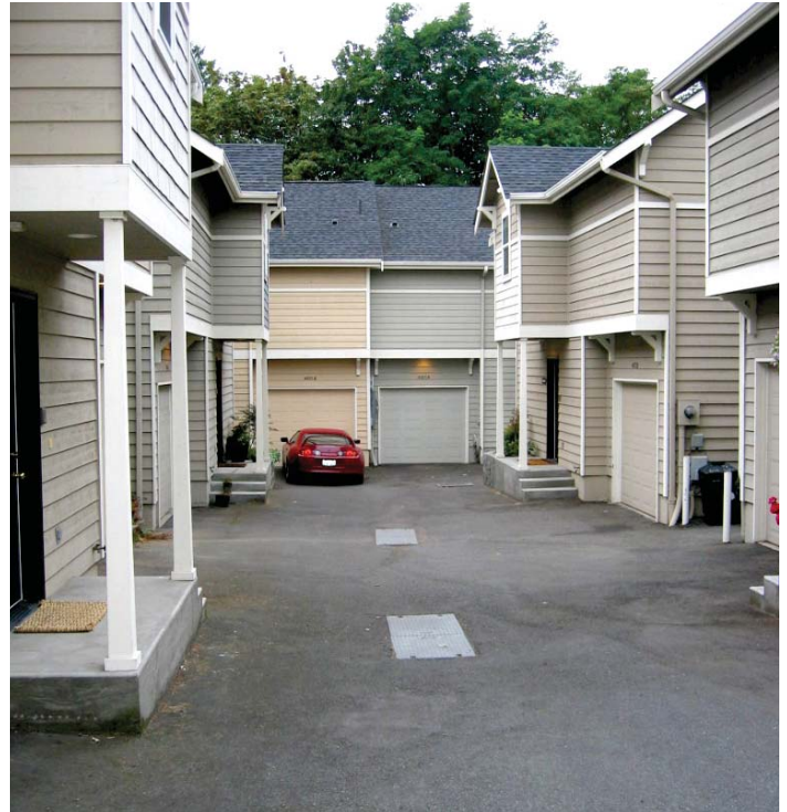
Fitting parking and driveways onto a site can pose difficult design challenges.
