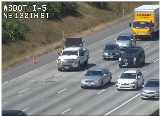
Figure 47. Pavement Buckling During the 2021 Heat Dome Event on Southbound I-5 at NE 130th St.
