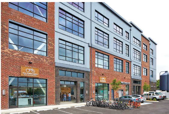
West Woodland Business Center, Ballard, WA. Photo by Aaron Locke, BCRA.
