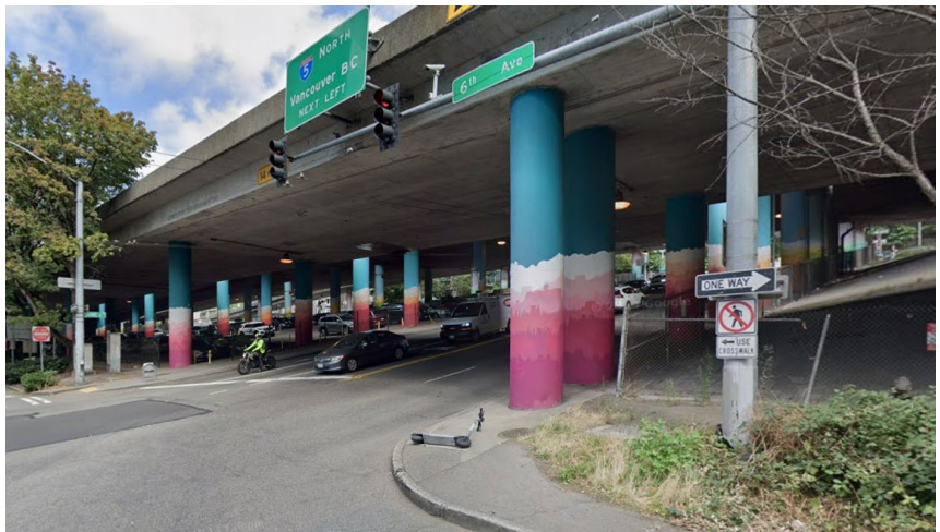
Cherry St I-5 Underpass
