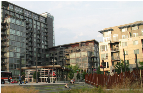
Placement minimized impacts to public park.
