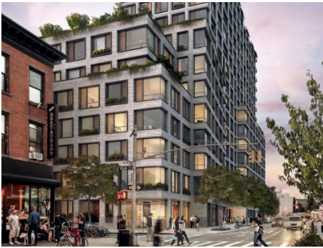
Transition to the adjacent townhouses.
