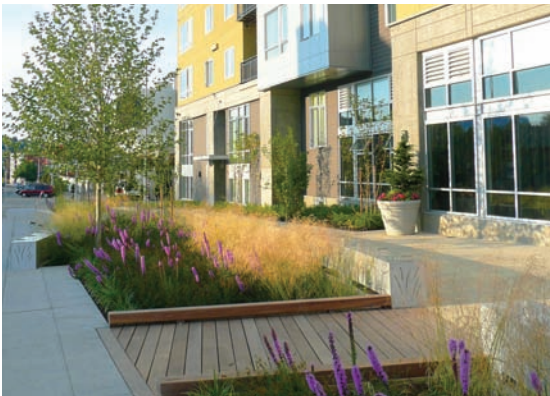
Rain gardens infiltrate stormwater runoff at Taylor 28, a new mixed-use multi-family housing project at the corner of Denny Way and Taylor Ave in SLU.
