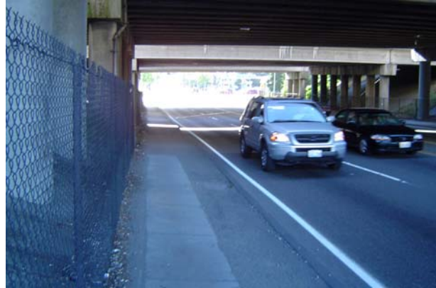
Freeway underpass Hostile to pedestrians
