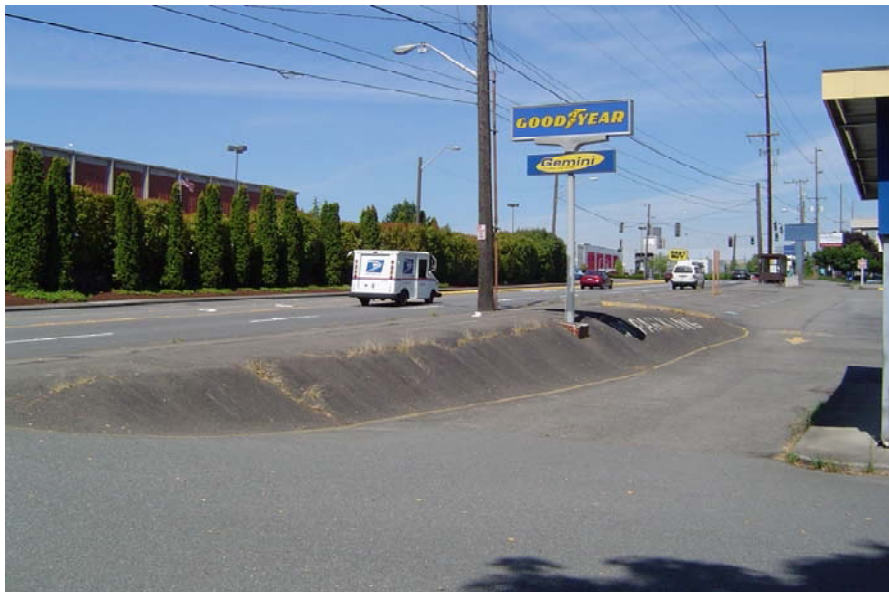
Site of Northgate Civic Center before construction of new park, branch library and community center and construction of 5 th Ave. NE Streetscape Improvements, Phase 1
