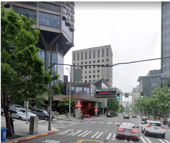
Seattle Municipal Tower with Ramp Opening
