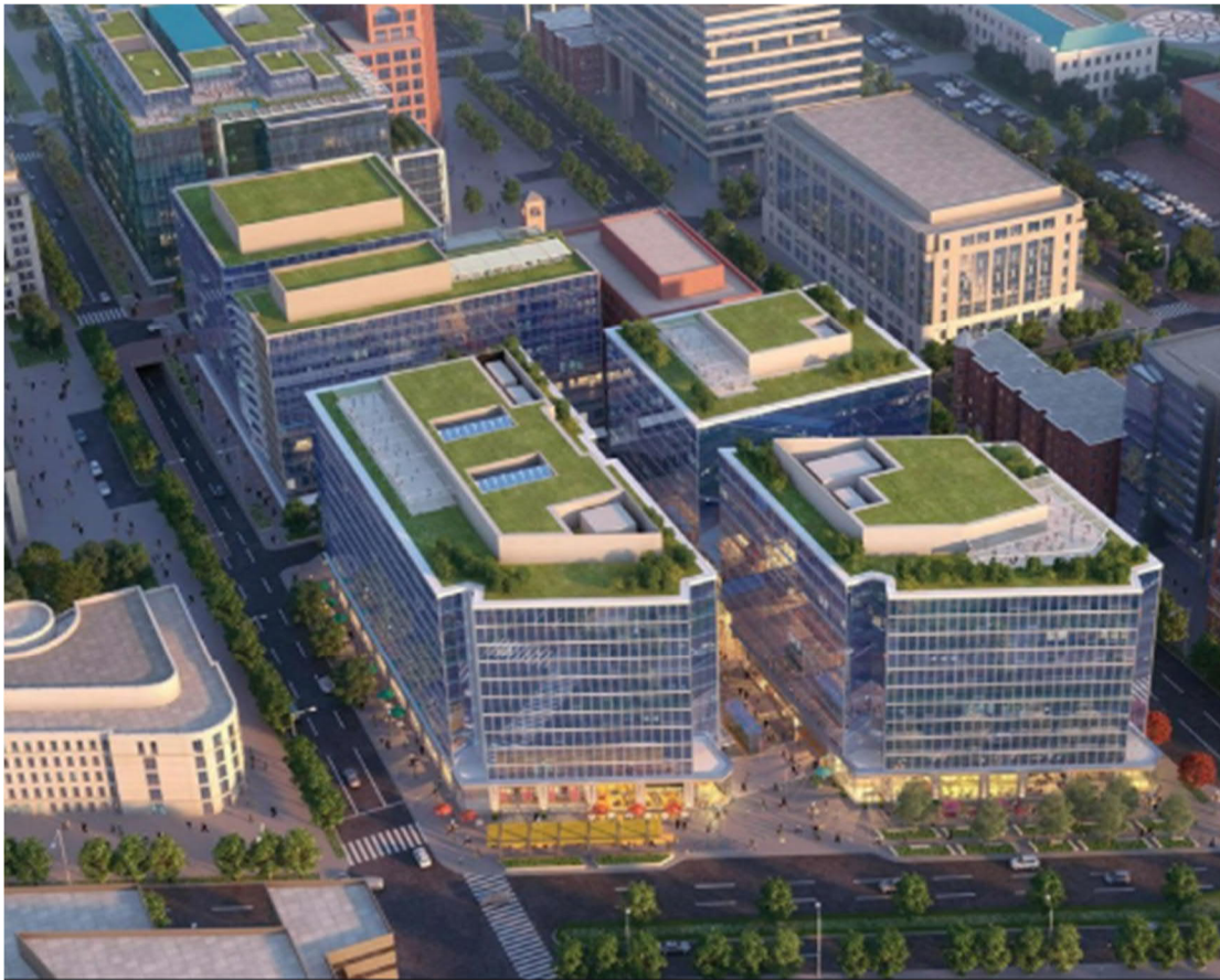
Capital Crossing Lid over the active I-395 freeway in Washington, D.C. Source: LERA structural engineers
