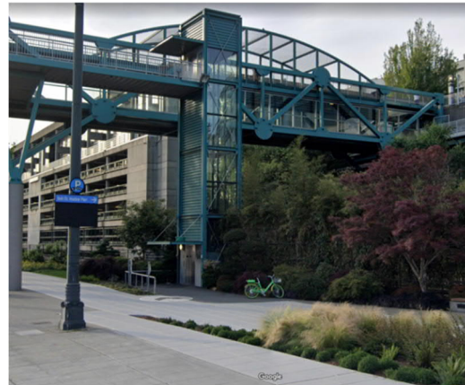
Bridge Connection on the Seattle Waterfront
