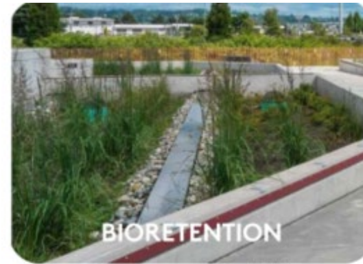
At Marysville Stormwater Park, WA
