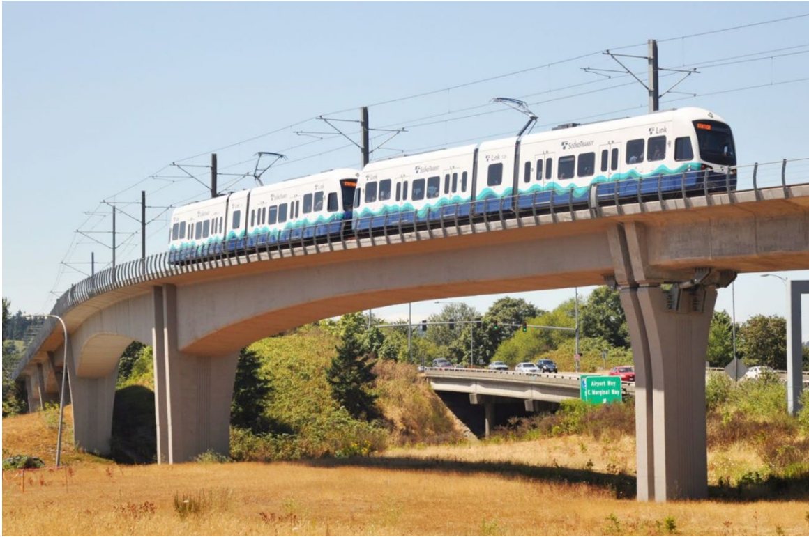
Balanced Cantilever Segmental Box Girder
