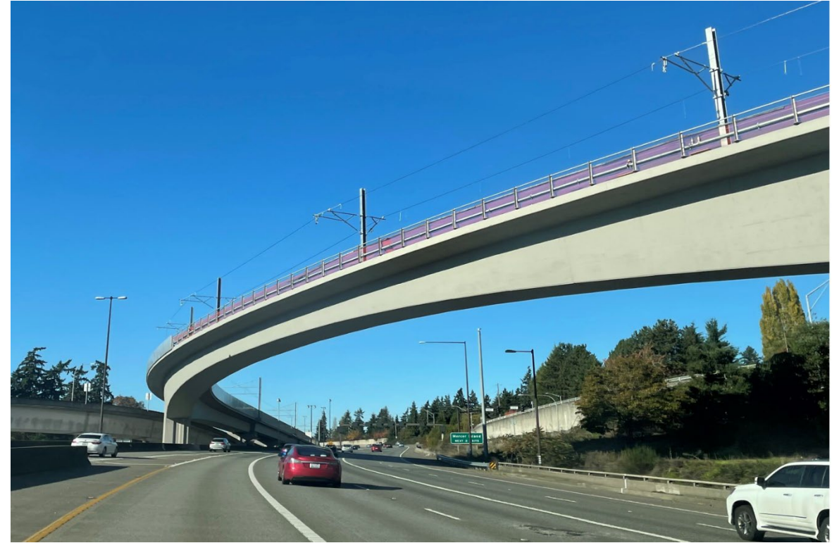
Balanced Cantilever Segmental Box Girder
