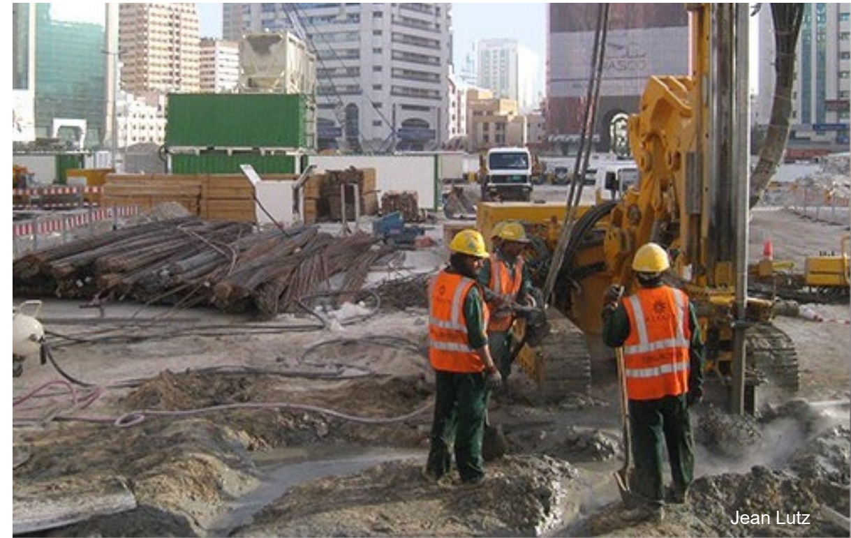
Ground Improvement (Jet Grouting)
