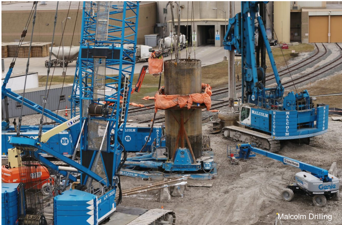
Drilled Shaft Installation
