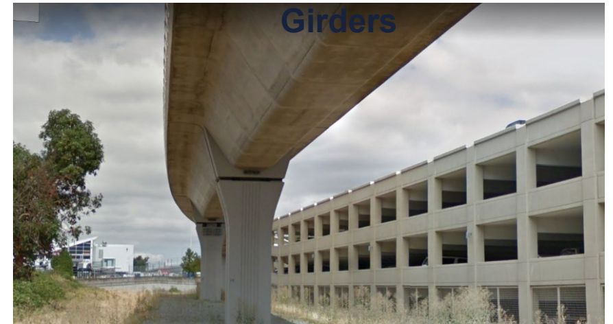
Post-Tensioned Box Girders
