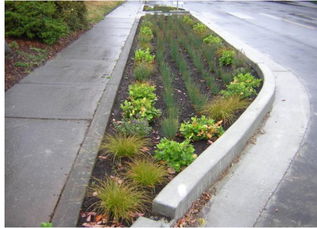
Figure 2: A typical rain garden
