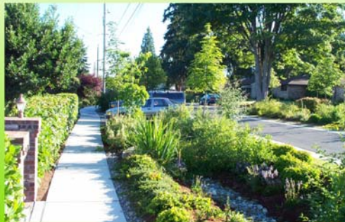
A landscaped swale and adjacent sidewalk on the SEA Street project.
