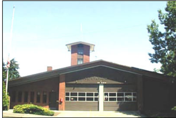
Fire Station 40: Seismic/Safety Remodel
