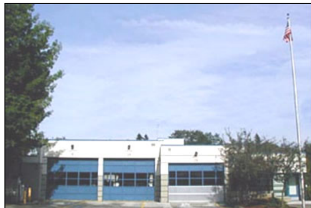
Fire Station 28: Major Renovation
