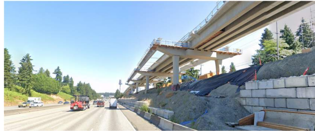
Construction progress as of Fall 2022
