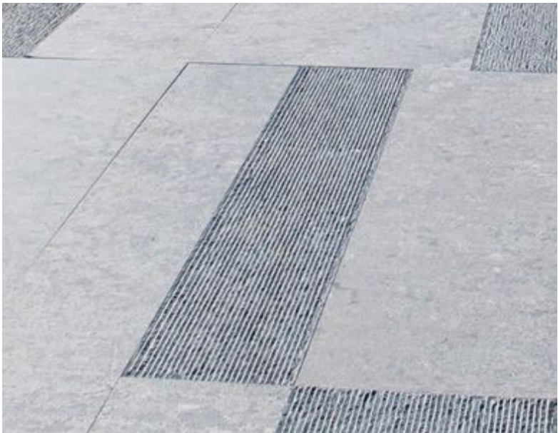
TINING TECHNIQUE IN CONCRETE
