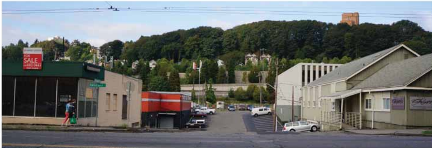
NORMAN STREET SUPPORT STRUCTURE - LOOKING WEST
