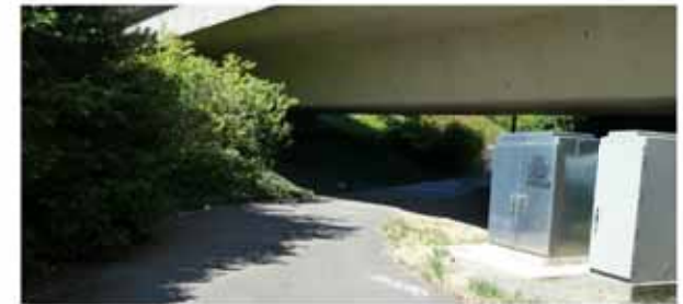
(C) MT. BAKER SUPPORT STRUCTURE - VIEW LOOKING NORTH
