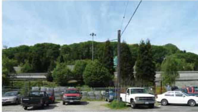
NORMAN STREET SUPPORT STRUCTURE - LOOKING WEST
