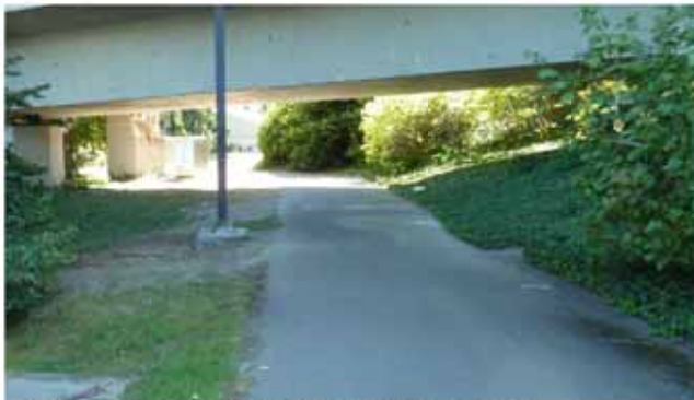
(A) MT. BAKER SUPPORT STRUCTURE - VIEW LOOKING SOUTH
