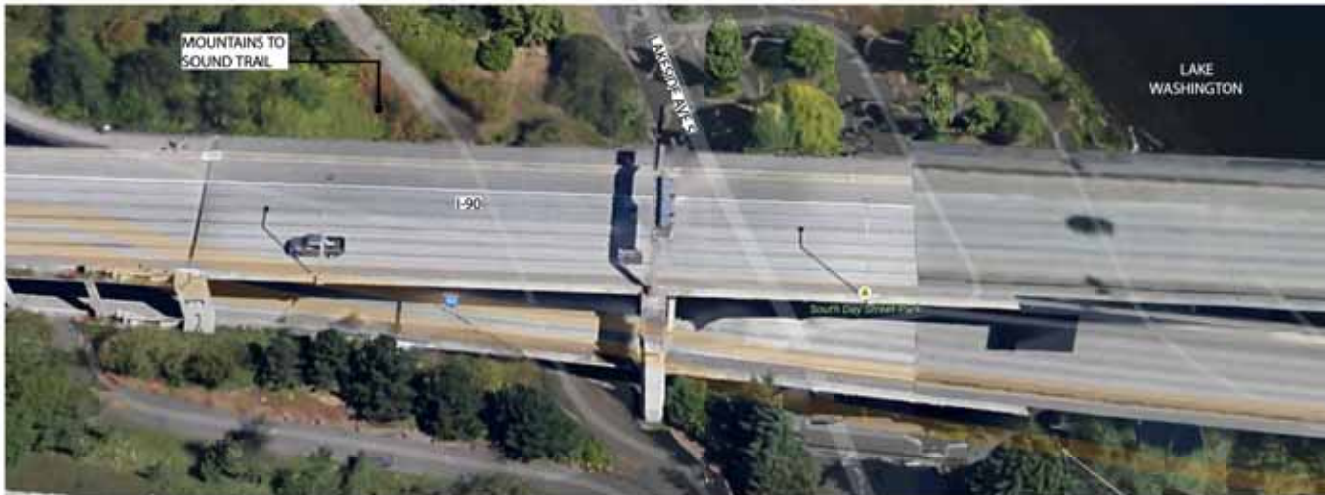
MT. BAKER SUPPORT STRUCTURE - AERIAL VIEW
