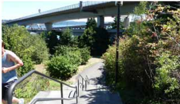
(B) MT. BAKER SUPPORT STRUCTURE - VIEW LOOKING SOUTH
