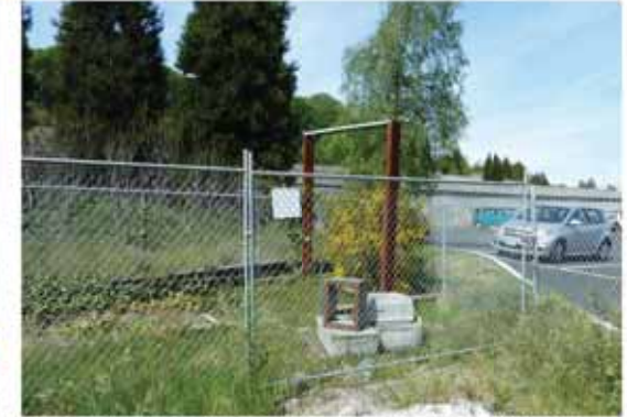
NORMAN STREET SUPPORT STRUCTURE - EXISTING CONDITIONS
