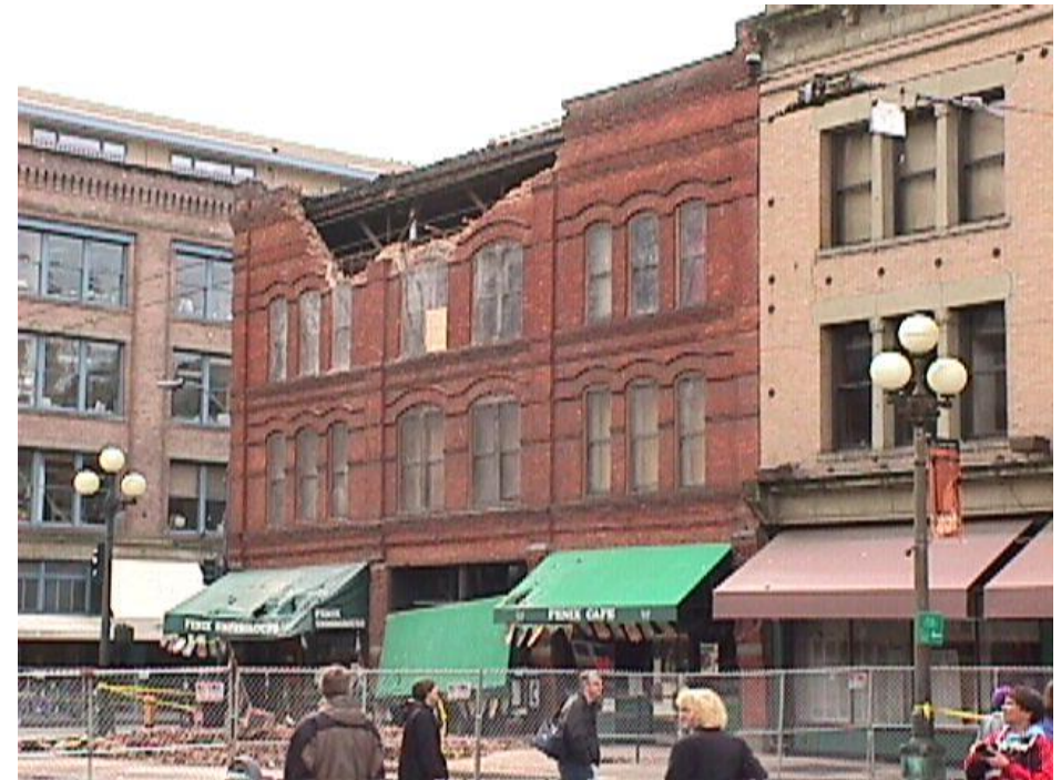
1999 Nisqually earthquake damage. USGS photo.
