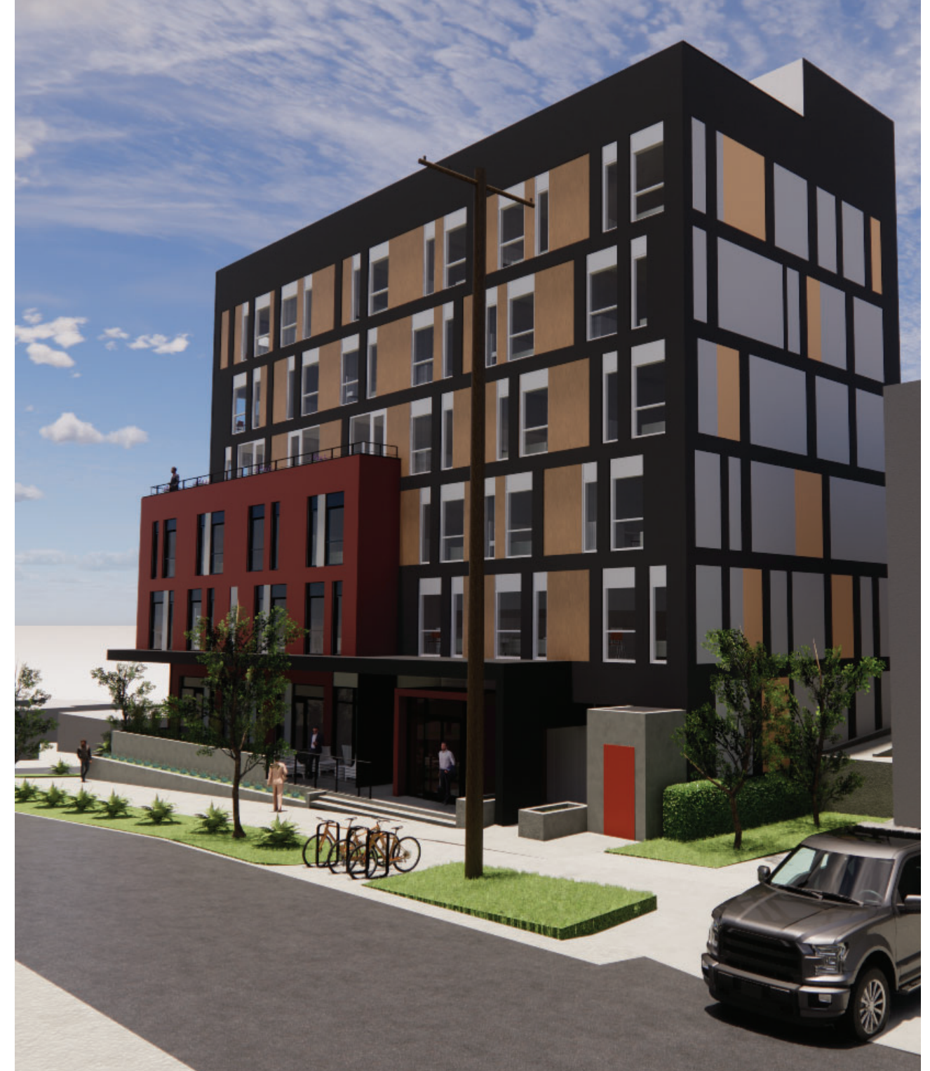
16TH AVE - LOOKING SOUTH
