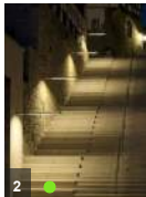
2 • Overhead lighting at exterior stairs
