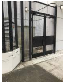
MAC service room door on Nagle Place
