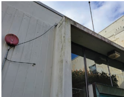
Stained concrete at window head
