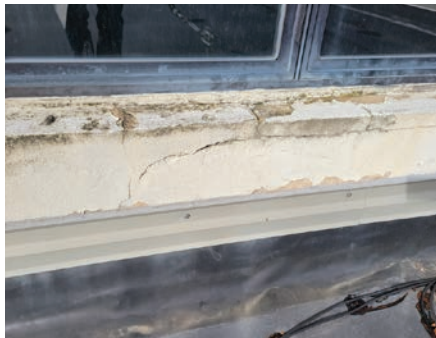
Concrete cracks
