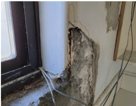
Uninsulated concrete interior
