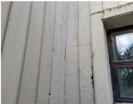
Failed sealant
