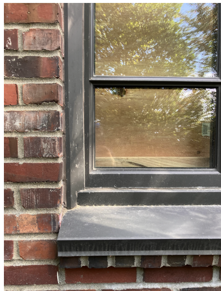
(E) Non-historical window section and photographs Wausau 8300i, Aluminum Casement Window, custom color True divided lite windows.
