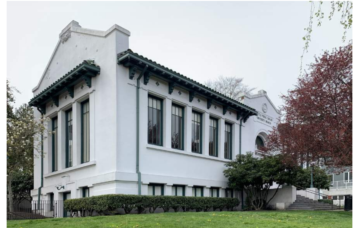
SOUTHEAST SITE + FACADE
