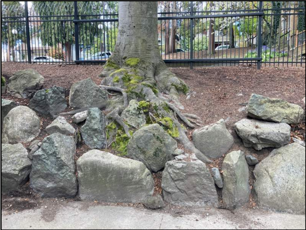
Photo 4. Roots from tree 283 that have become intertwined in the existing rockery
