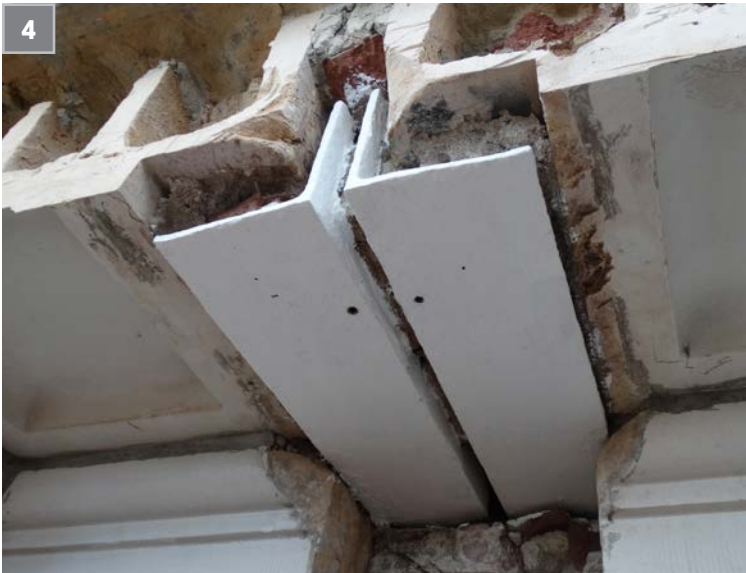
1. TERRA COTTA SPALL, PREVIOUSLY PATCHED AND HAS FAILED AGAIN
