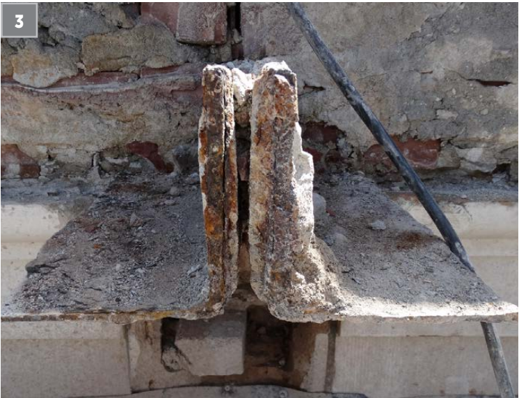
3. EXAMPLE OF CORRODED SUPPORT STEEL WITH EXCESSIVE LOSS AND NEEDING REPLACEMENT.
