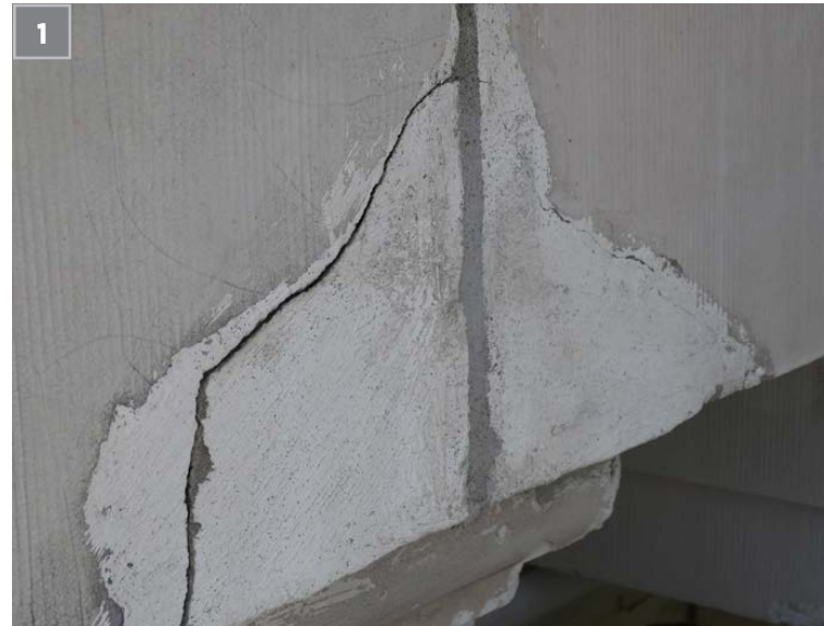
1. TERRA COTTA SPALL, PREVIOUSLY PATCHED AND HAS FAILED AGAIN
