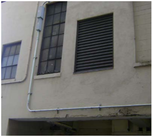
4 Exposed Non-Original Conduit and Mechanical Equipment Broken, Painted Windows
