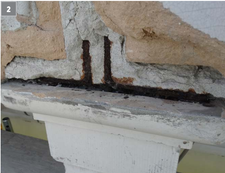
2. OXIDE JACKING AT SUPPORT STEEL CAUSING THE FAILED PATCH IN PHOTO 1
