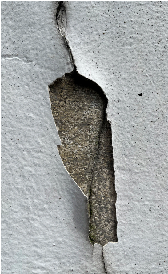
TYPICAL BANDING; PAINT OVER CEMENTITIOUS BLOCK
