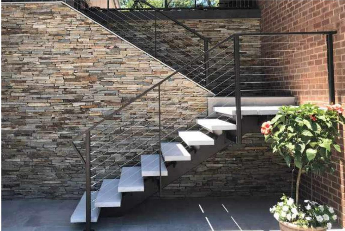
CABLE RAILING HANDRAIL AT FLOATING STAIRS
