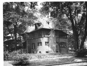
N—Exterior Plaster to the Ground. No Underpinning shows in this House
